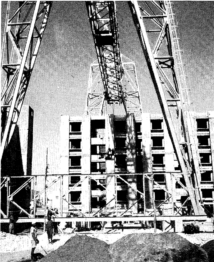
. . . and for structural strength.
